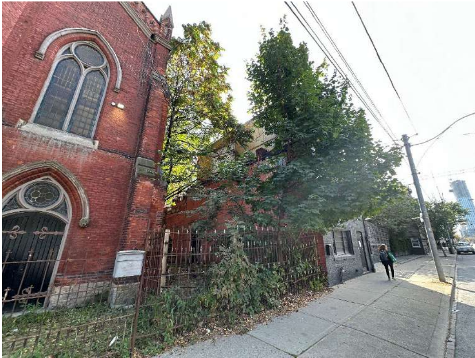
Subject Property – North Elevation Along Queen Street East
