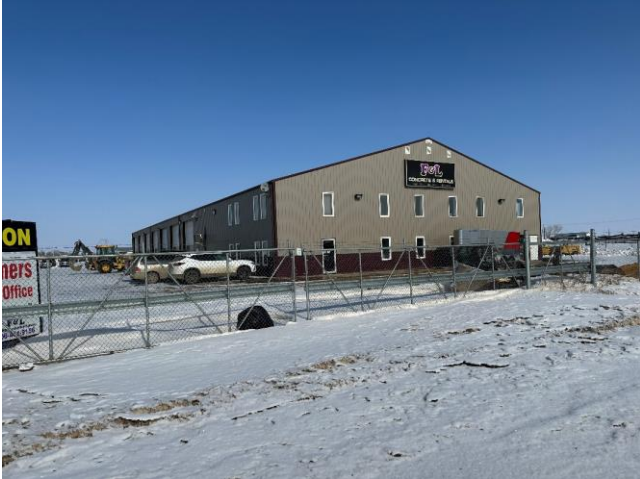
1) Main Office and Shop East (front) and South Sides
