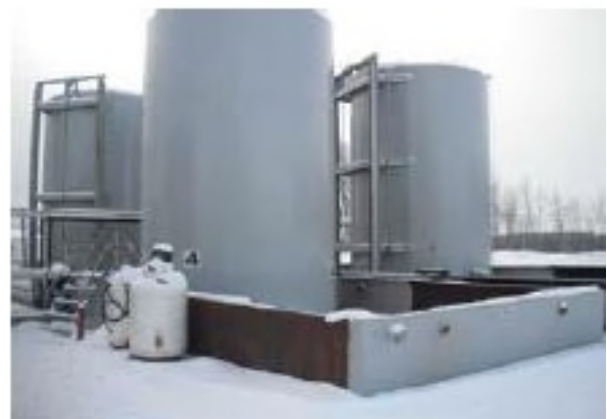
Steel Spill Containment System
