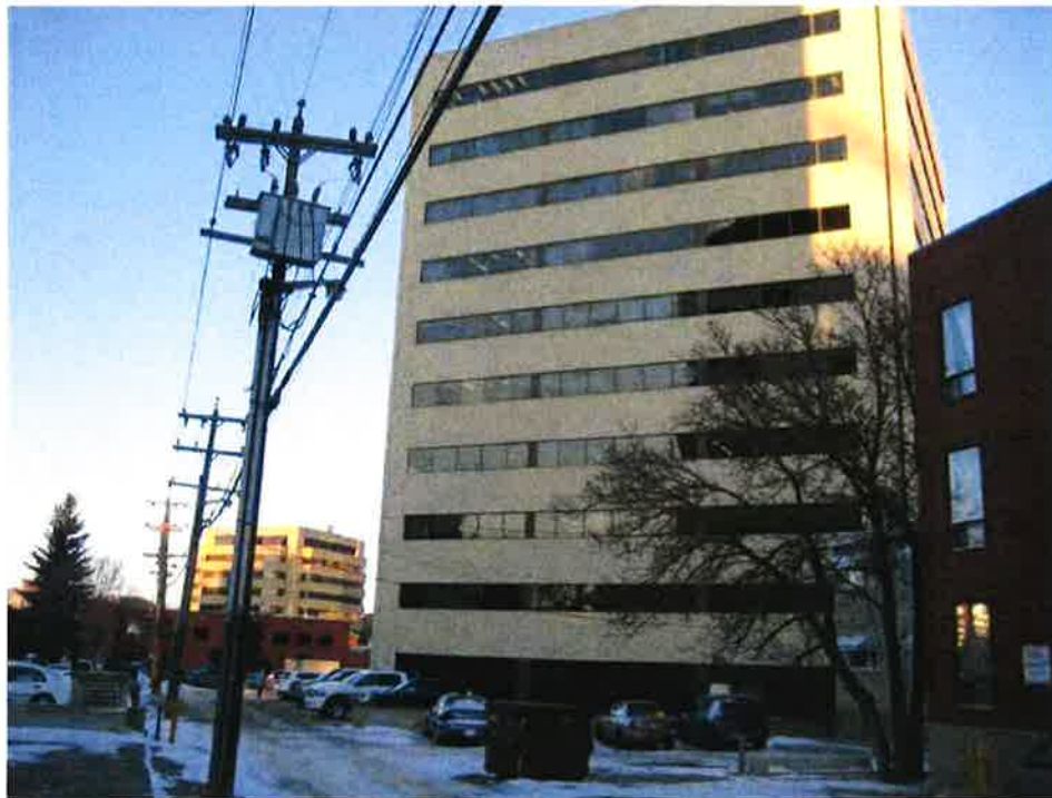
Photo 2: Southwest building elevation
