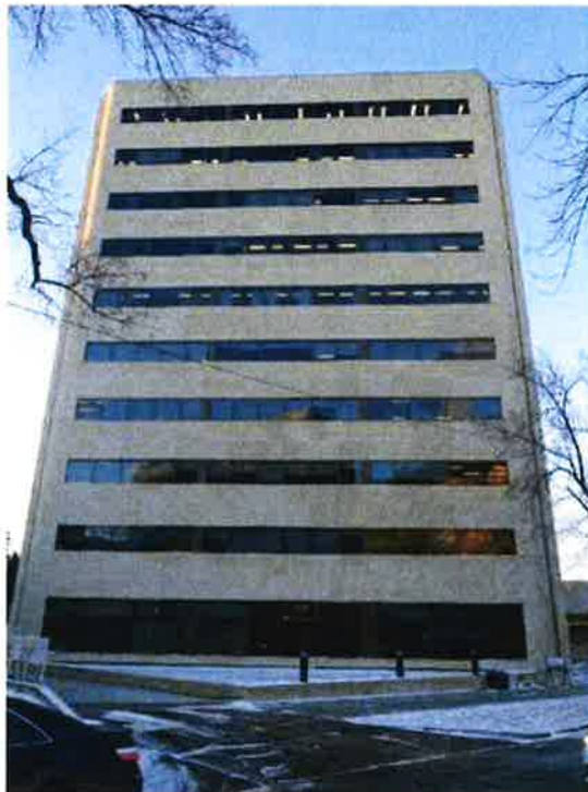
Photo 4: Overview of tower viewed from southeast
