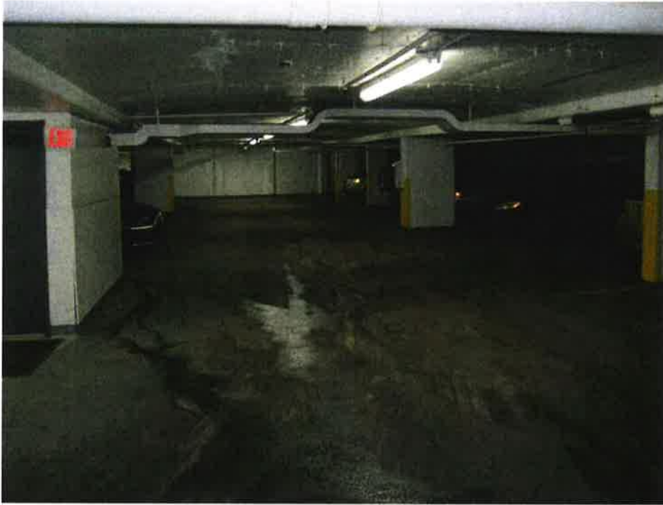
Photo 7: Typical parking level
