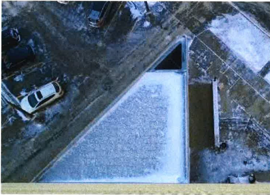
Photo 5: Overview of lower level roof (Zone 3)
