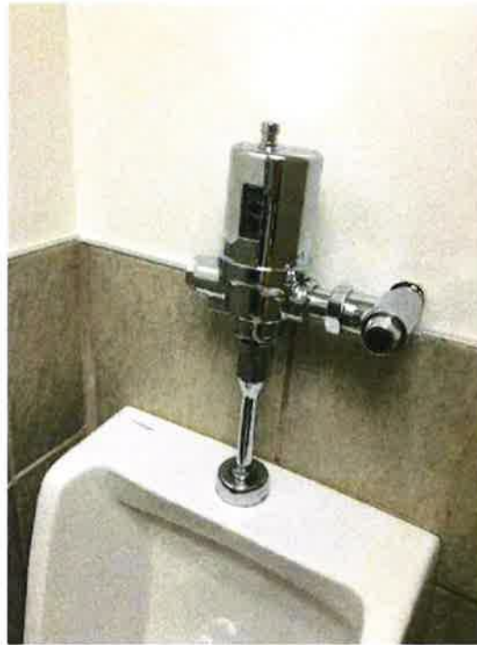
Photo 2: Typical automatic flush valve urinal
