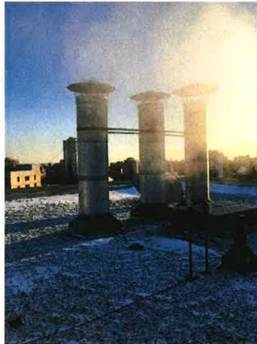
Photo 120: Roof - boiler flues
