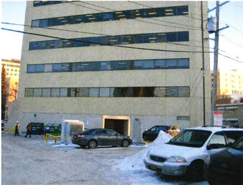
Photo 3: Northwest elevation – loading dock area
