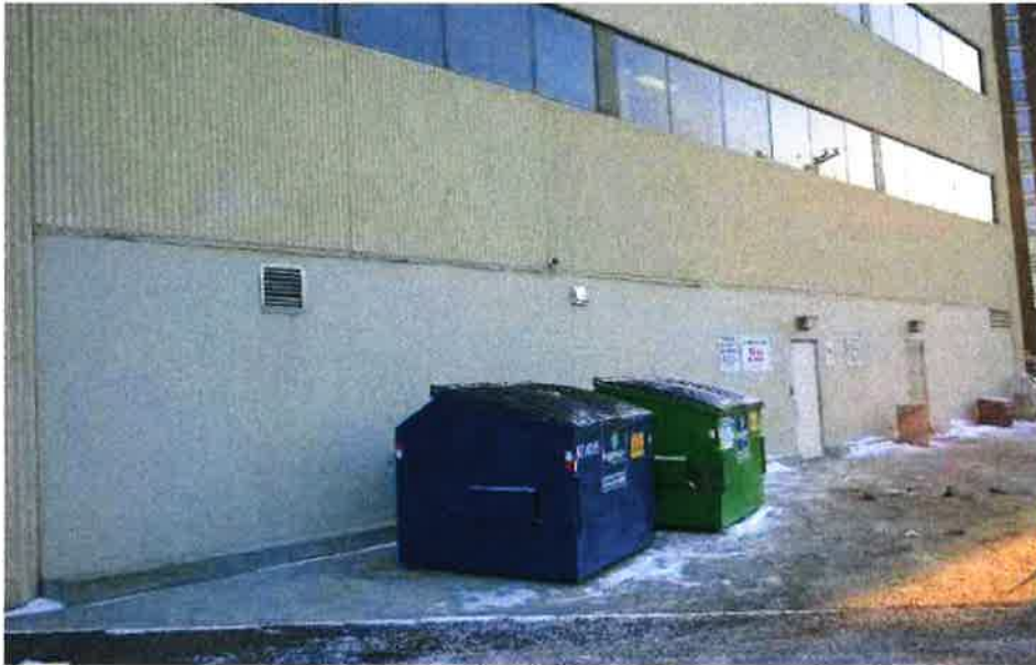
Photo 5: Block wall on northwest elevation
