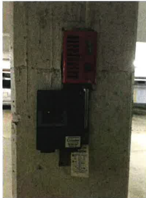
Photo 112: Parkade gas detector
