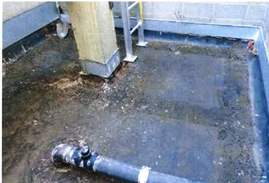
Photo 4: Overview of Cooling Tower Roof (Zone 2A)
