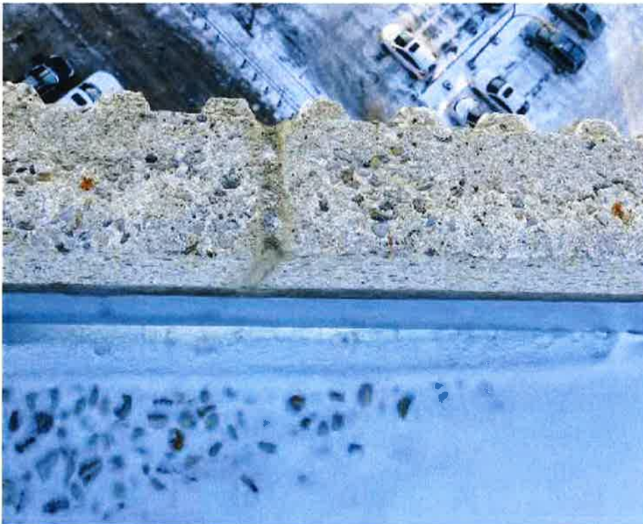
Photo 10: Close up of caulked joints at typical parapet location
