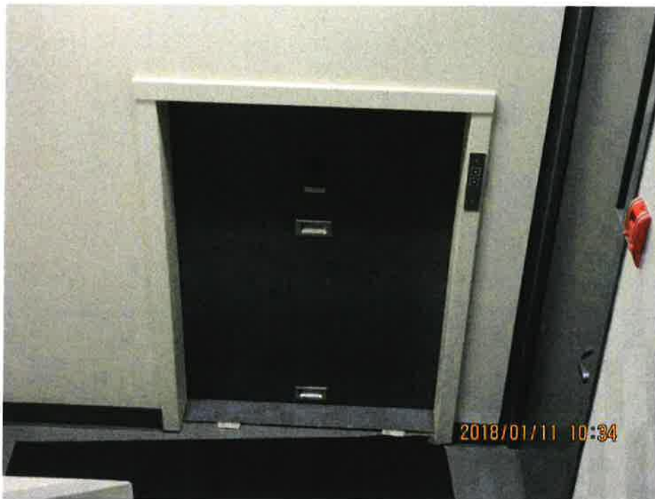
Photo 22: Typical entrance assembly (Dumbwaiter 5)
