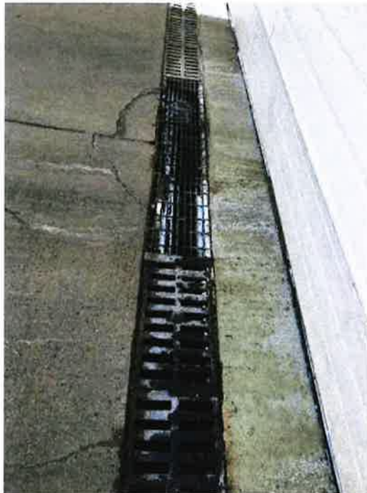
Photo 130: Trench drain at bottom of entrance ramp
