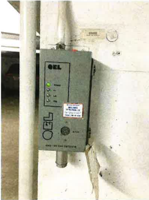
Photo 115: Parkade gas detector
