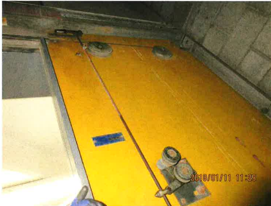
Photo 13: Hall interlock assembly (Parkade 4)
