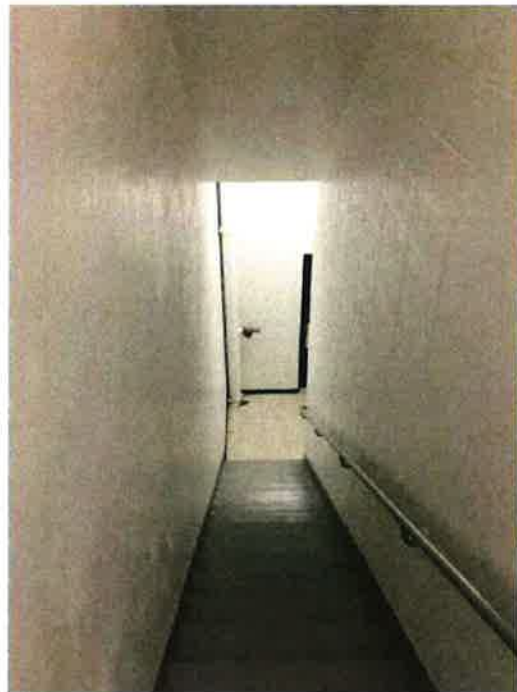
Photo 118: Top of stairwell, showing standpipe
