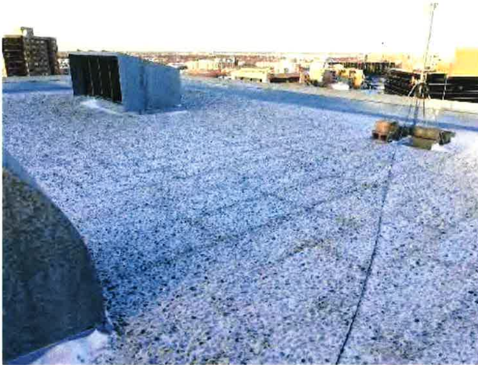
Photo 1: Overview of main roof (Zone 1)
