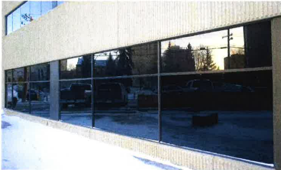
Photo 7: Typical ground floor windows
