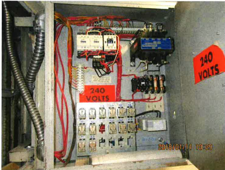
Photo 19: Controller (Dumbwaiter 5)
