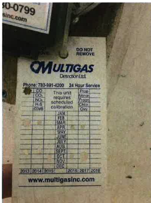
Photo 113: Gas detector service tag
