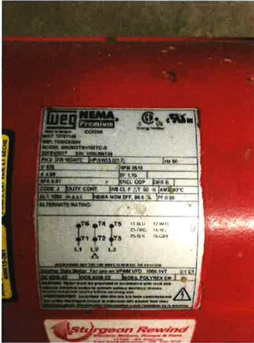
Photo 91: Primary domestic cold water pump motor tag
