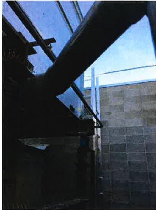
Photo 63: Cooling tower access ladder
