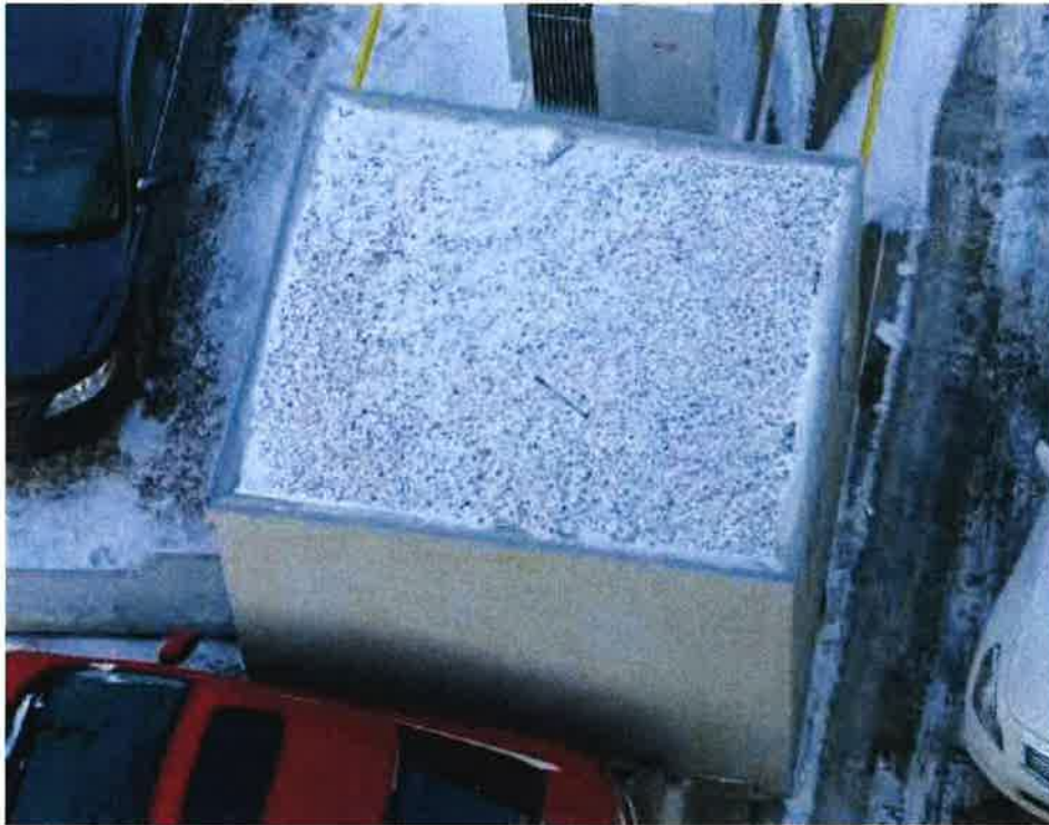
Photo 7: Overview of Mechanical Doghouse Roof (Zone 5)
