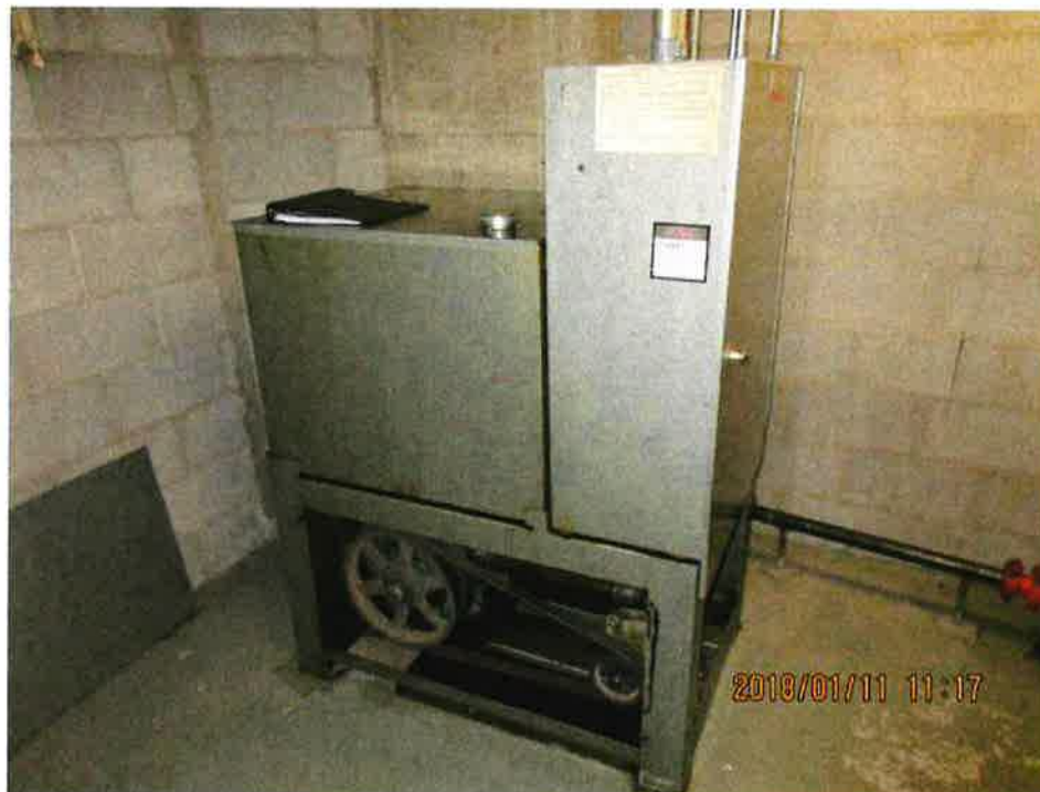
Photo 10: Power unit assembly (Parkade 4)
