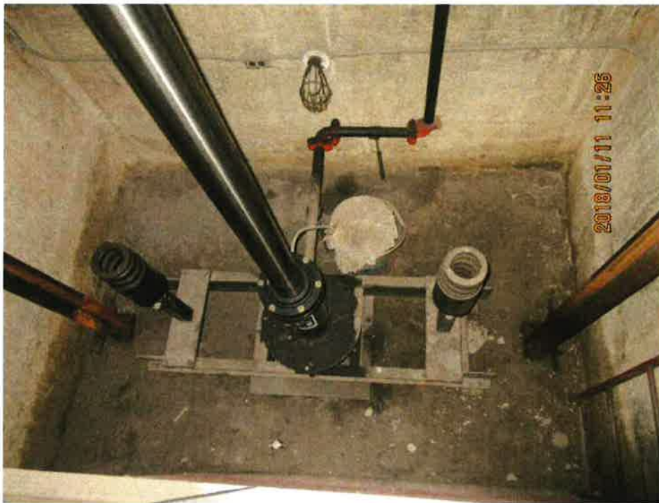
Photo 14: Pit area (Parkade 4)
