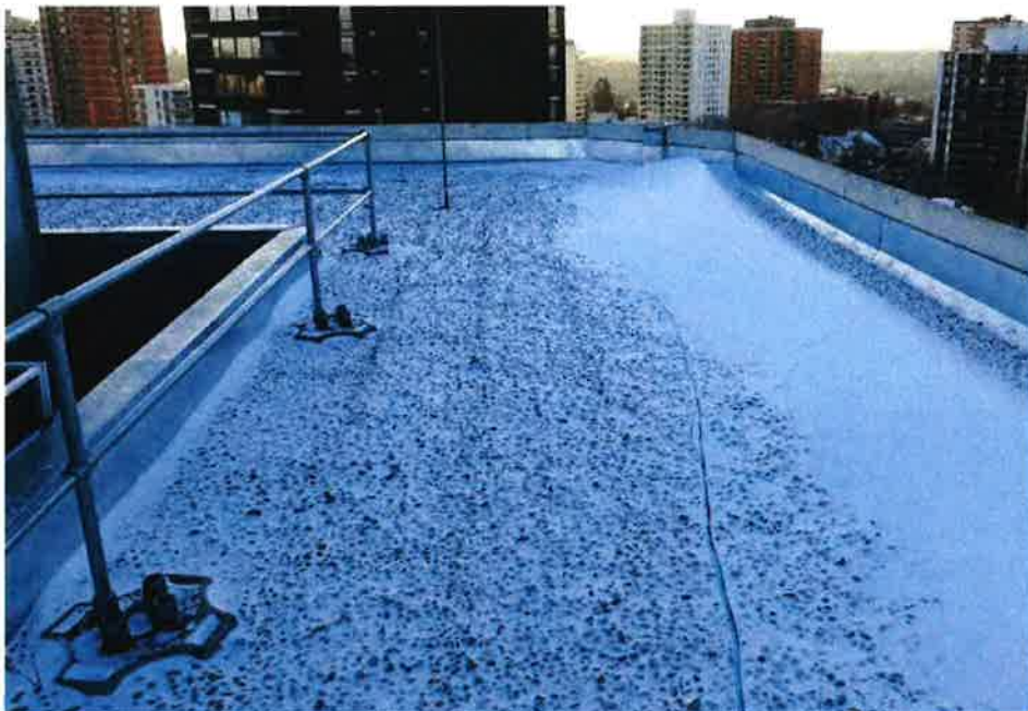
Photo 2: Overview of main roof (Zone 1)
