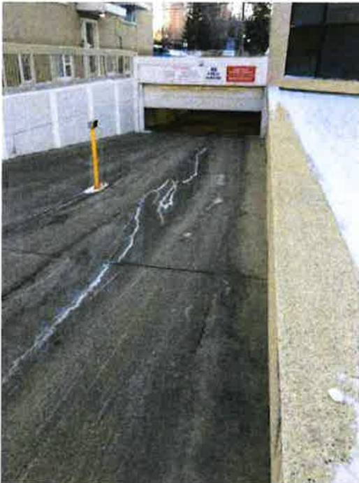
Photo 129: Parkade entrance ramp
