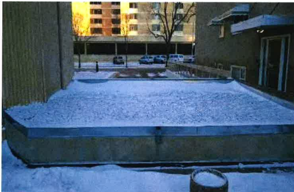
Photo 6: Overview of parking garage ramp roof (Zone 4)
