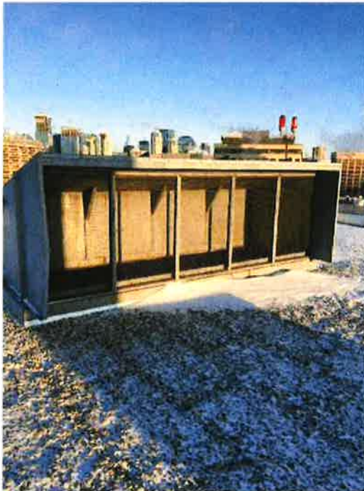
Photo 119: Roof - AHU air intake
