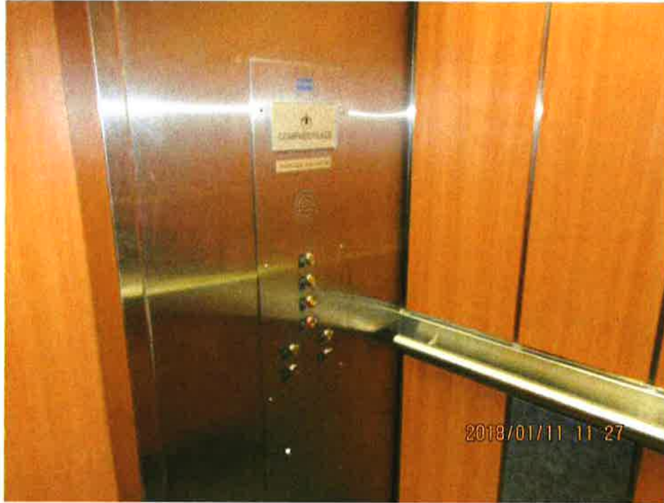
Photo 15: Car fixtures (Parkade 4)
