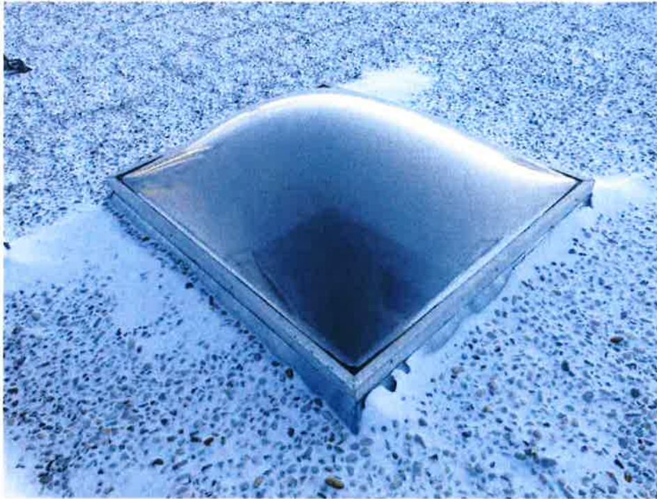
Photo 3: Overview of skylight on main roof
