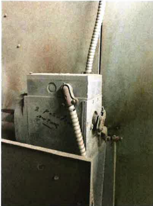
Photo 84: MAU noted as 2-speed motor
