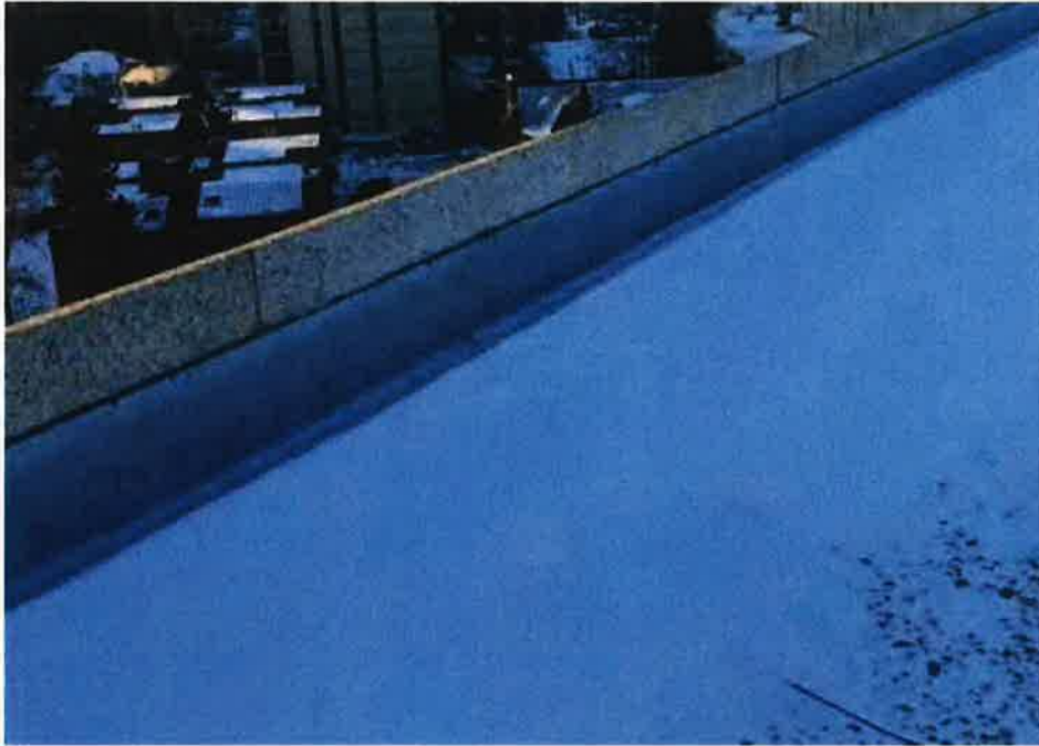
Photo 9: Caulking along top of counter flashing on main tower roof
