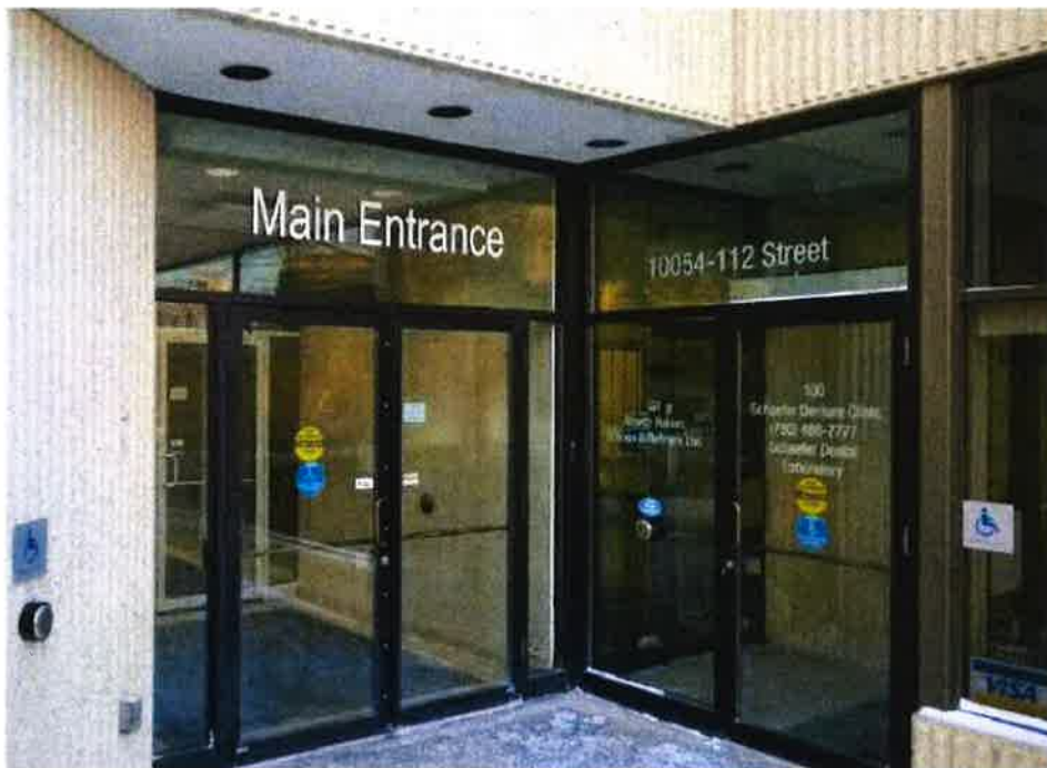
Photo 6: Building entrance system on northeast side of building
