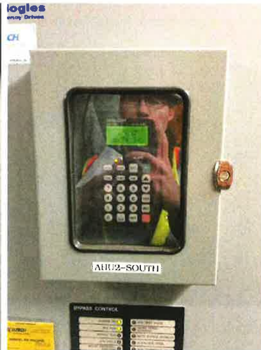
Photo 44: AHU2 VFD
