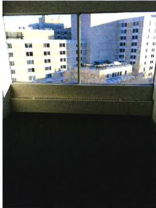
Photo 71: Perimeter heating
