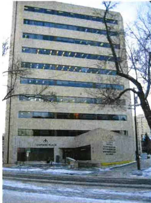
Photo 1: Northeast building elevation
