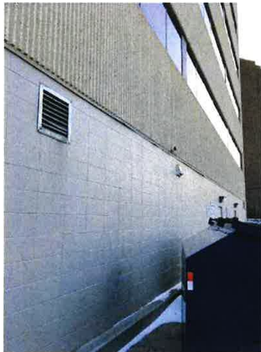
Photo 126: Exhaust outlets and louvres, backside of building
