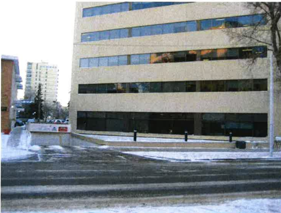
Photo 4: Southeast corner – entrance to parking structure
