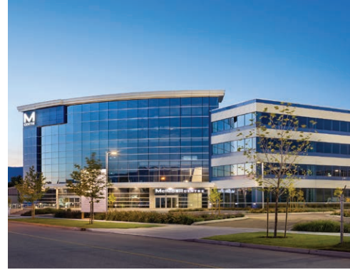
2300 LECKIE ROAD KELOWNA | 78,000 SF Office Building SOLD 2016
