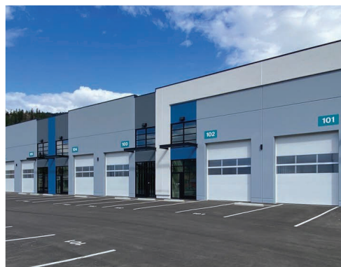
BUILDING 1 2648 KYLE RD WEST KELOWNA | 34,575 SF Multi-Unit Industrial Building SOLD Q4 2021
