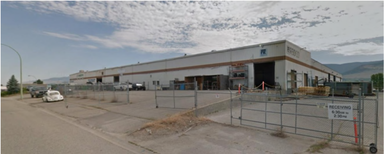
555 Adams Rd west facing (shown here without new exterior cladding)
