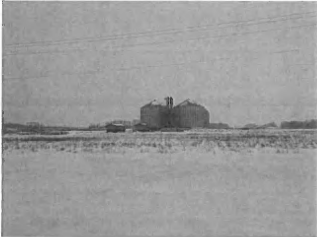
Bins – north side, view from street
