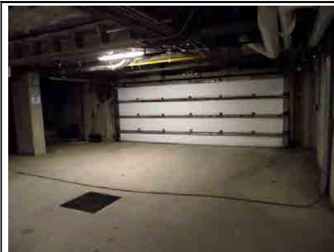
UNDERGROUND PARKING GARAGE
