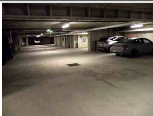
UNDERGROUND PARKING GARAGE
