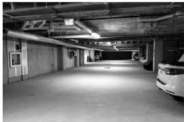
View of Underground Parking
