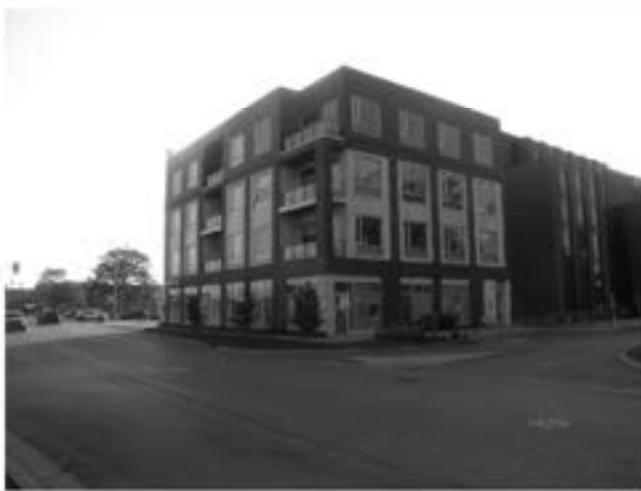
Rear and North Elevation
