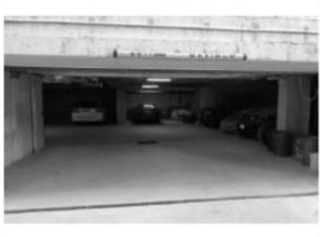
View of Underground Parking
