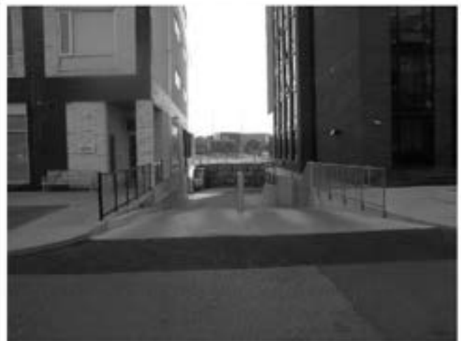
View of Parking Garage Ramp
