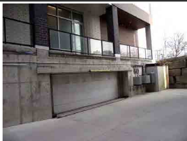
UNDERGROUND PARKING GARAGE
