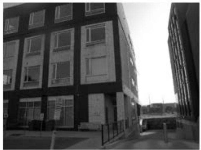
South Elevation and Parking Garage Ramp
